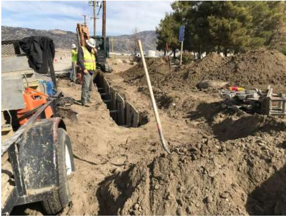
Figure 3 – The final section of 12 kV underground conduit was installed along Pellisier Road.
