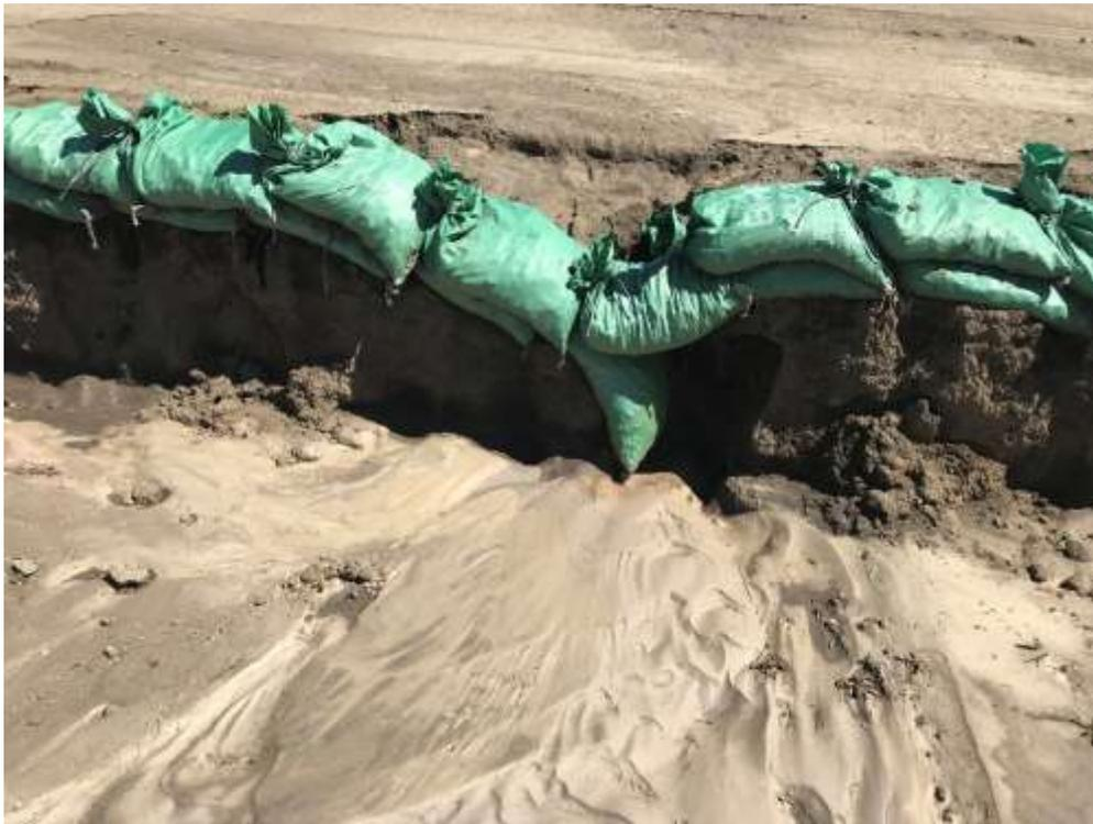
Figure 5 – Run-on from adjacent farm land occurred during a storm event. A discrepancy between the elevation of the adjacent farm field and the substation channel feature is being evaluated by SCE to avoid this becoming a continual problem.
