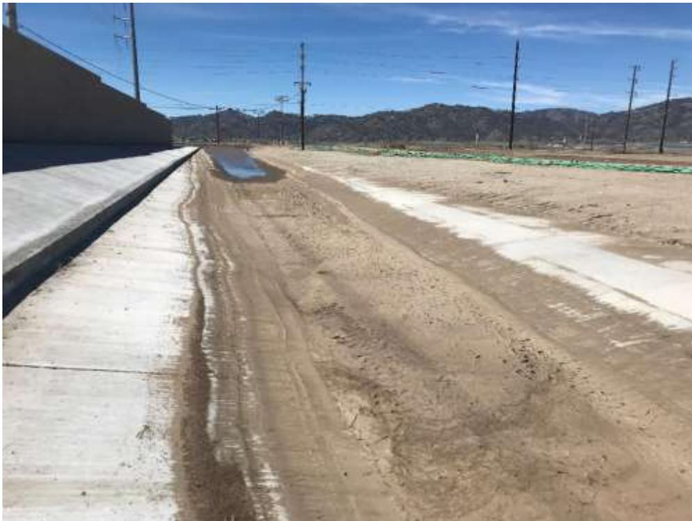
Figure 6 – Run-on from the adjacent farming operations. Sediment collected in the perimeter concrete channel.
