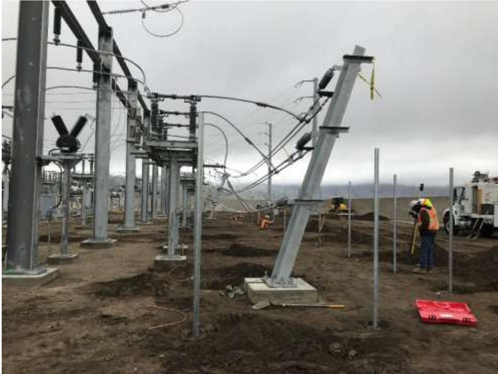
Figure 1 – H&M crew installing fencing and jumpers on the 66 kV rack.
