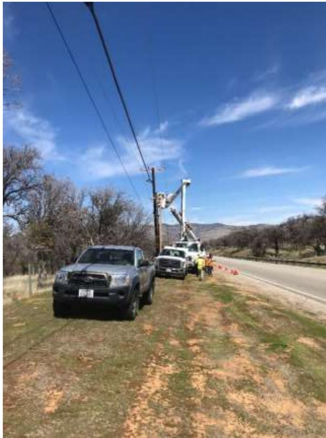
Figure 4 – H&M crews conducting pole replacement along Highway 202.
