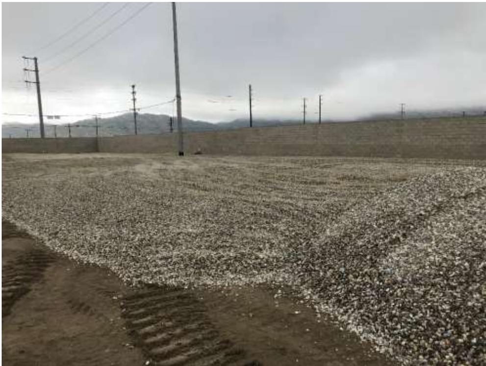
Figure 2 – Civil work including final grading and rock placement at the Banducci Substation.
