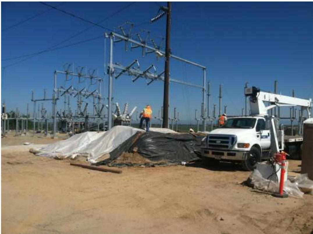
Figure 3 – Crews continue to maintain soil stockpile coverings and other SWPPP BMPs. View northeast, 03/19/15.
