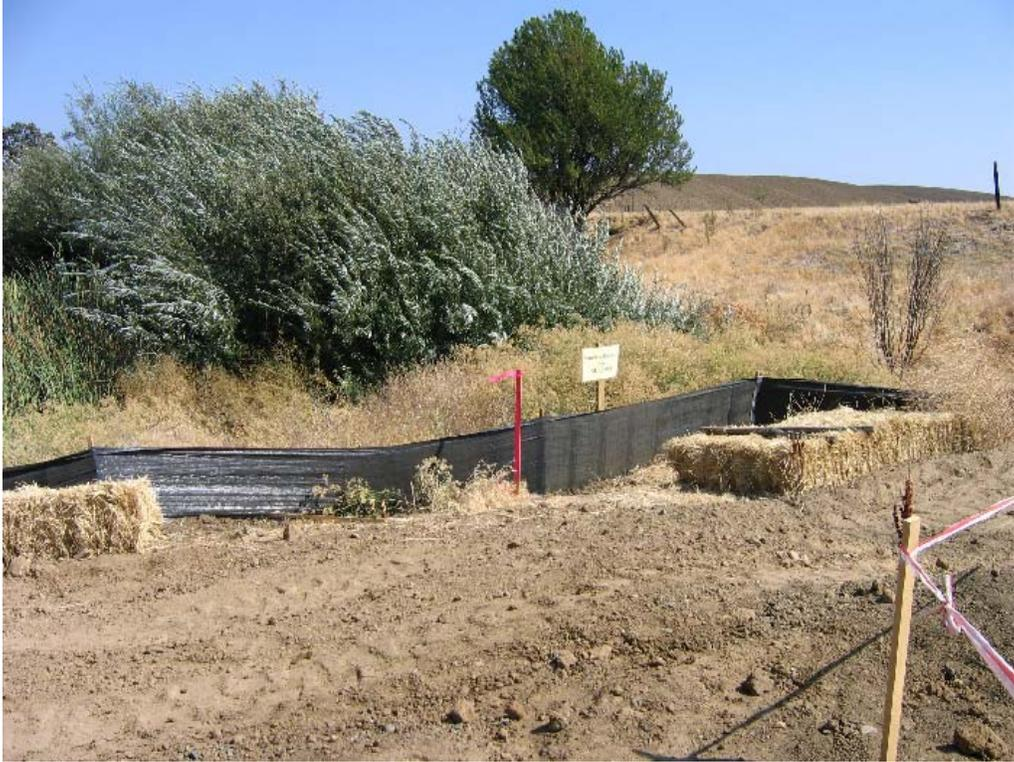
**Figure 3** – Silt fences and other erosion controls in place near Sand Creek.
