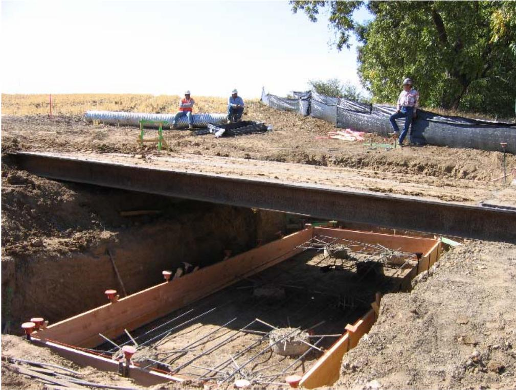
**Figure 1** – Bridge foundation work on south side of Sand Creek.
