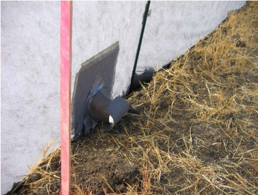
**Figure 4** – One-way escape funnel installed in wildlife exclusion fencing around substation site, October 3, 2007.
