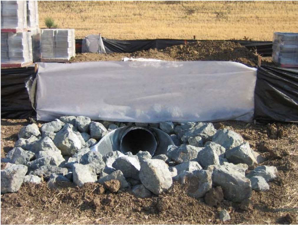
**Figure 3** – New culvert installed along access road at wetland area #4, October 25, 2007.
