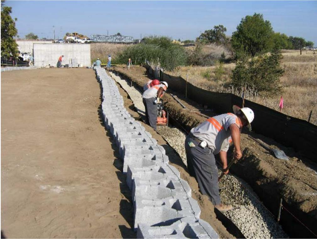
**Figure 1** – Crews working on keystone retaining wall on the south side of Sand Creek, October 25, 2007.
