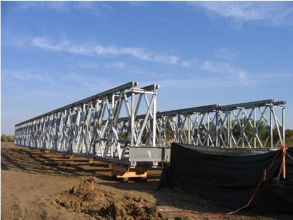
**Figure 2** – Bridge structure at staging area waiting to be set on bridge foundations , October 25, 2007.
