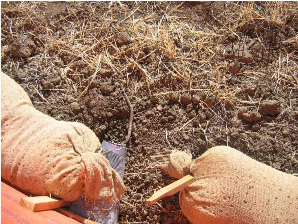
**Figure 2** – Juvenile gopher snake using the escape funnel installed in the wildlife exclusion fence along the access road, November 14, 2007.
