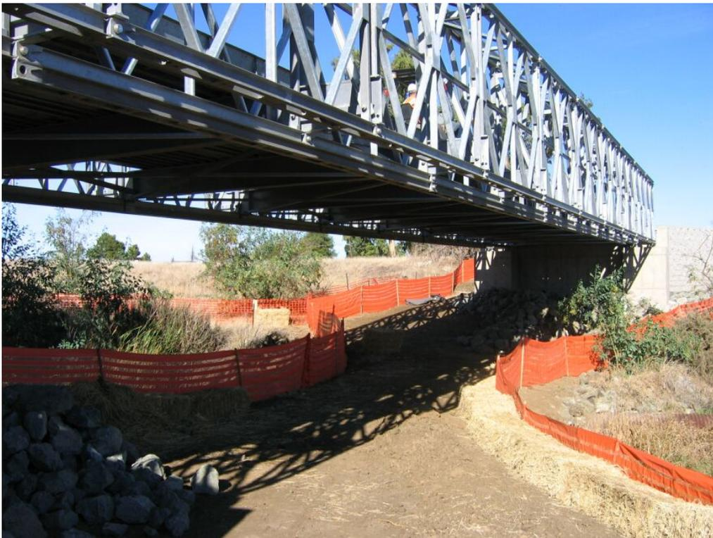
**Figure 4** – Erosion controls added under bridge over Sand Creek, November 14, 2007.
