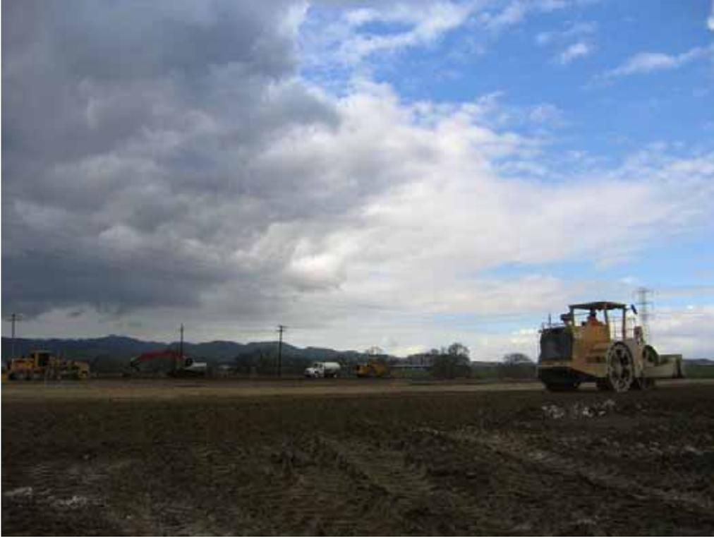
**Figure 1** – Grading and compacting lime treated soil at the substation site, February 22, 2008.
