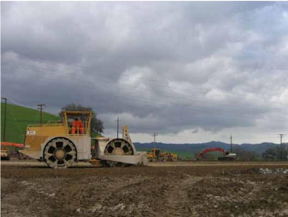
**Figure 2** – Grading and compacting lime treated soil at the substation, February 22, 2008.
