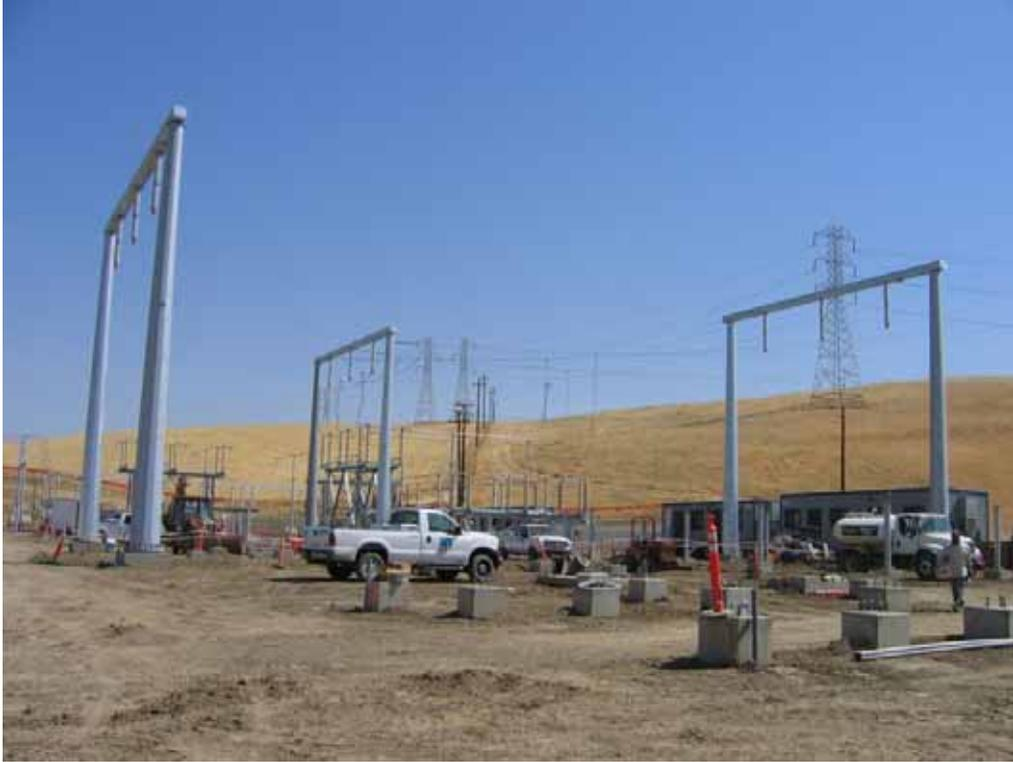
**Figure 2** – Bus structures being installed for Phase 2 and 3 at substation site, June 13, 2008.
