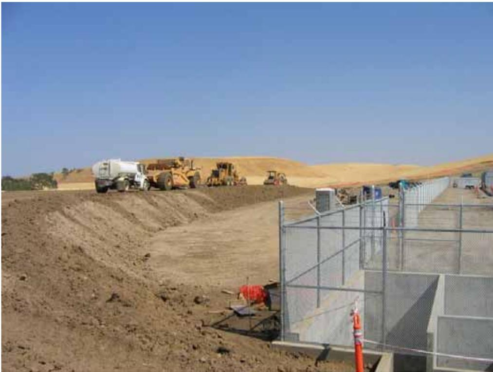
**Figure 3** – Earthen berm being built up around the outside of the substation, June 13, 2008.
