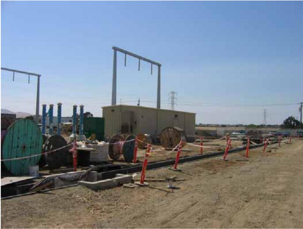
**Figure 1** – Electrical cable trays installed in the ground at substation site, June 13, 2008.
