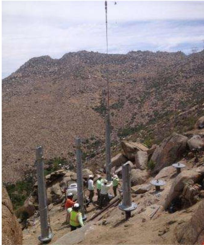
Figure 3. Permanent platform assembly at Tower 1044.
