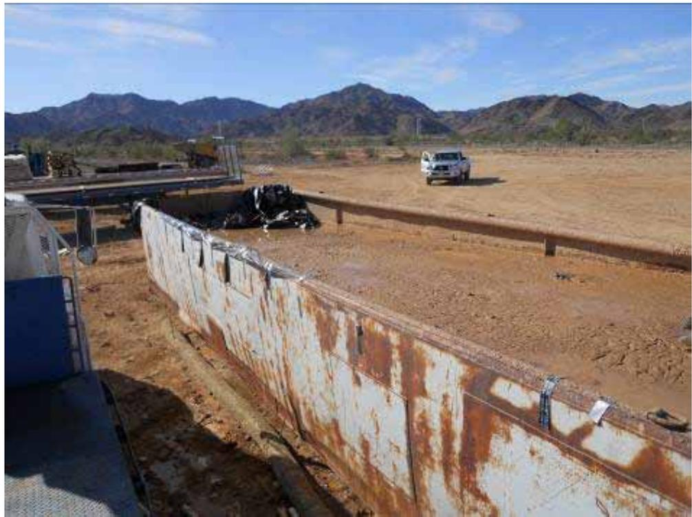
**Figure 6:** Mud tank with pooled surface water left uncovered at Red Bluff Substation.
