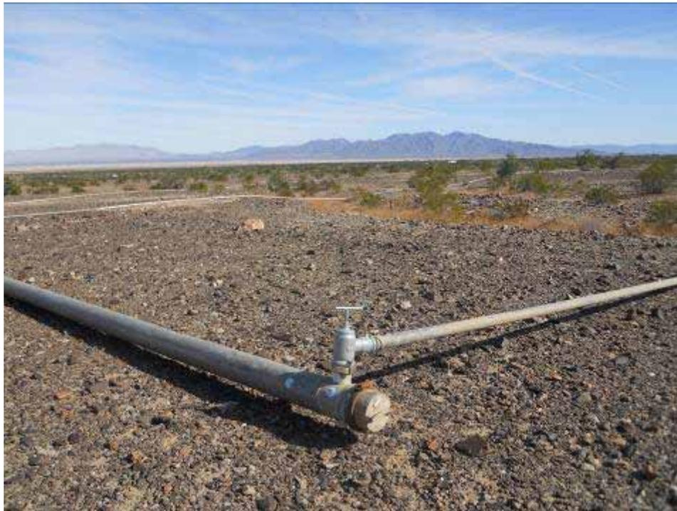
**Figure 4:** Sprinkler system installed at Red Bluff Substation site to control water well release flows.
