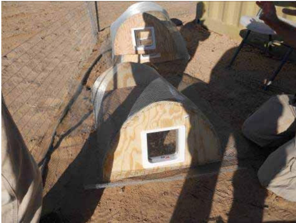
**Figure 3:** Structures designed by SCE kit fox biologists to exclude kit foxes from active burrows at CRS site.
