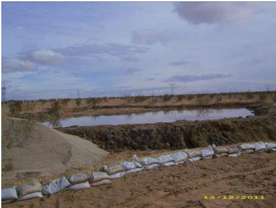
**Figure 6:** Earthen berm constructed to contain drill cuttings at the Red Bluff Substation site.
