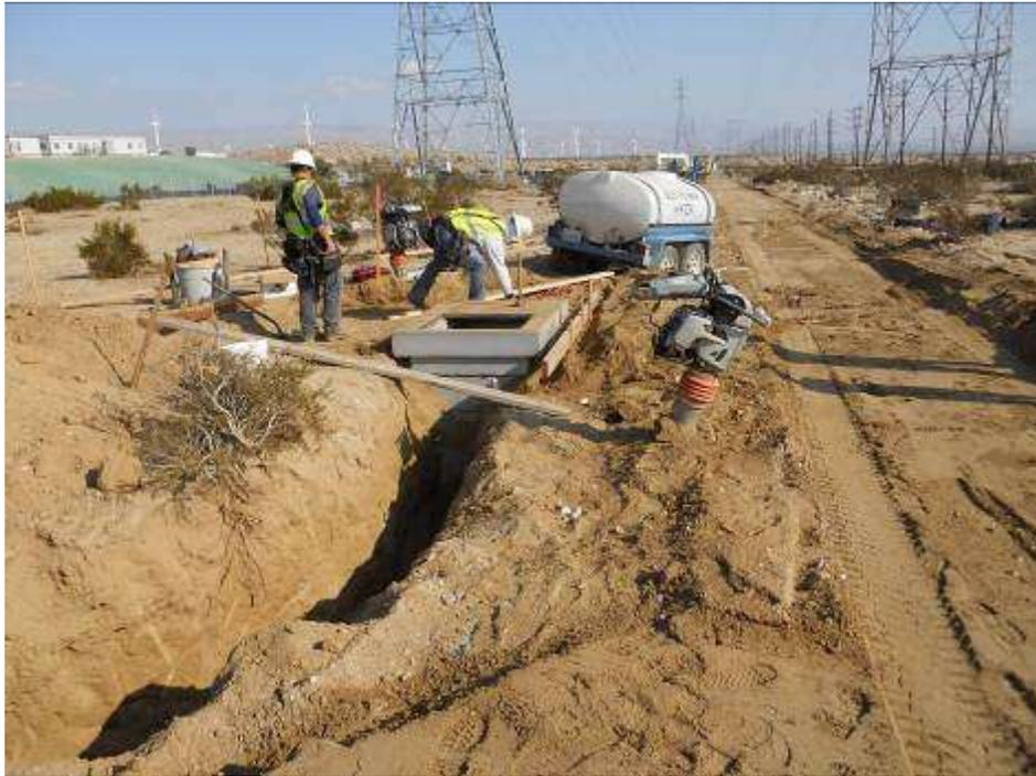
**Figure 1:** Construction of a pull box site along the underground power alignment for the Devers #1 Construction Yard.
