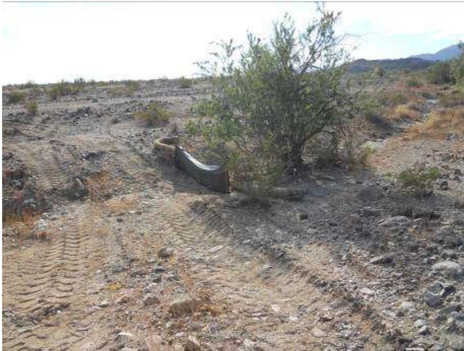
**Figure 7:** BMPs installed along drainage in anticipation of 24-hour well testing activities at the Red Bluff Substation site.
