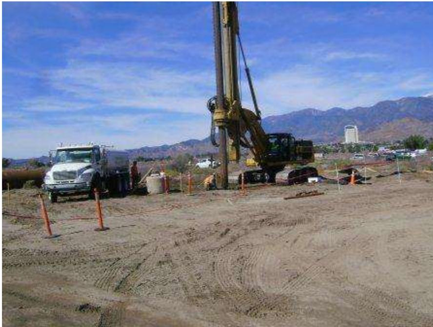
**Figure 4.** Foundation drilling at Tower R1.
