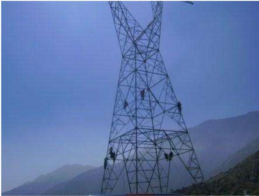
**Figure 3.** Tower assembly (crews backbolting) at Tower 1057.
