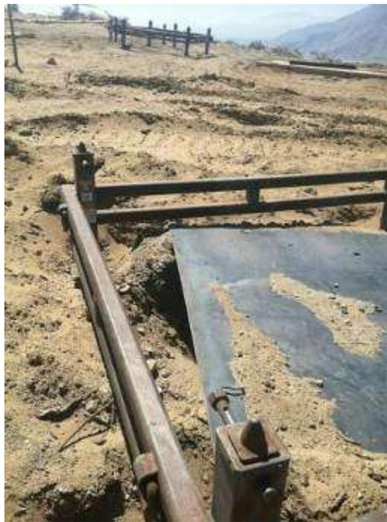
**Figure 4.** Foundation excavation inadequately covered at Tower 1015 (Photo taken from FRED Incident Report).
