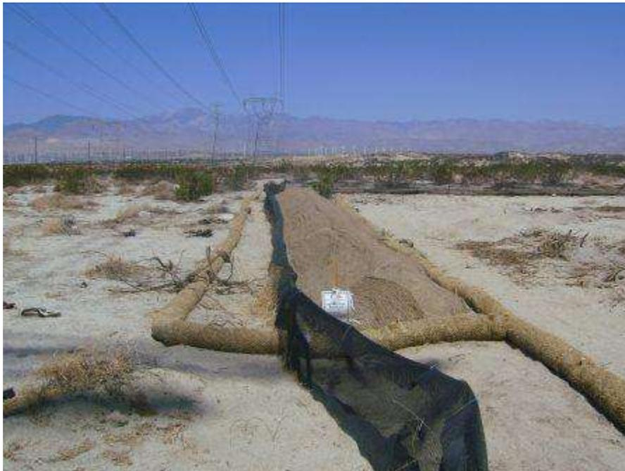
**Figure 6.** Topsoil salvage at Tower 2016.
