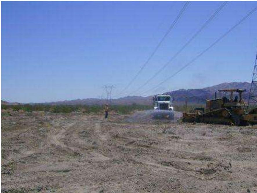
**Figure 2.** Crane pad grading at Tower 2335.
