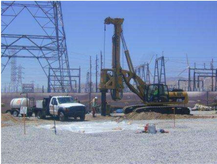
**Figure 5.** Foundation excavation at Tower 1001. Tower 1001 is within the Devers 1 Yard.
