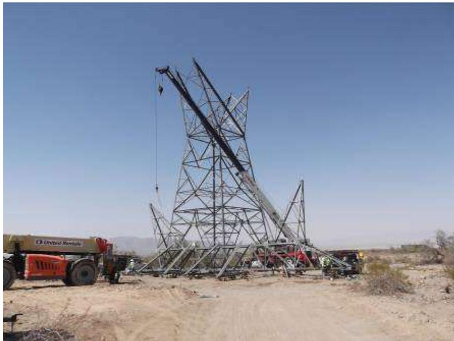
**Figure 4.** Tower assembly at Tower RB1-3E.
