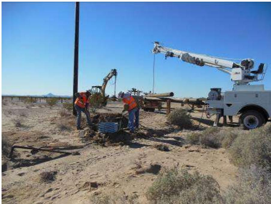
Figure 6. Hole excavation for wooden pole installation along the Southeast Telecommunication Route.
