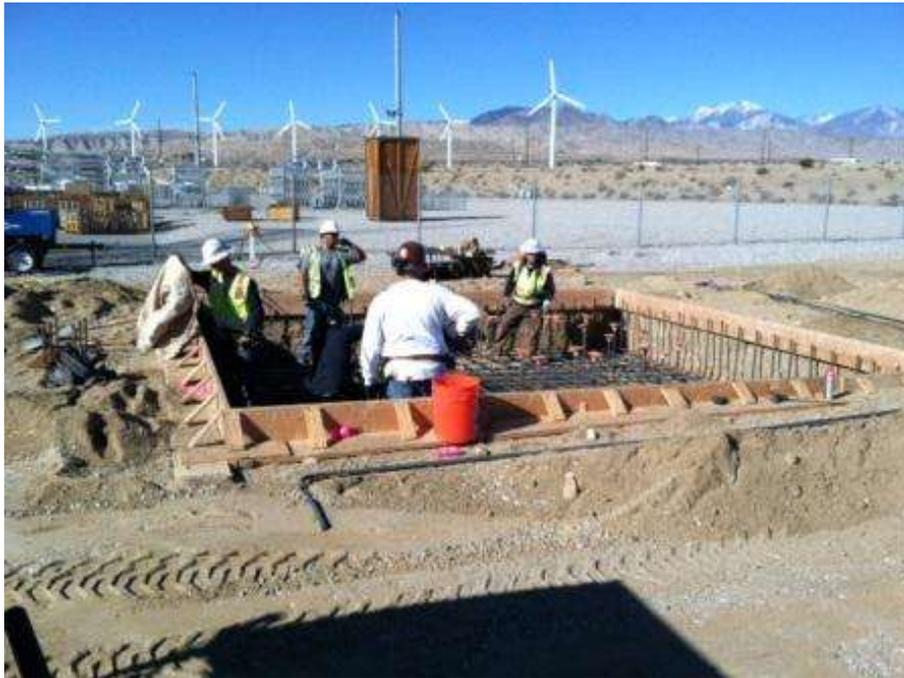
Figure 8. Foundation work within the Devers Substation.
