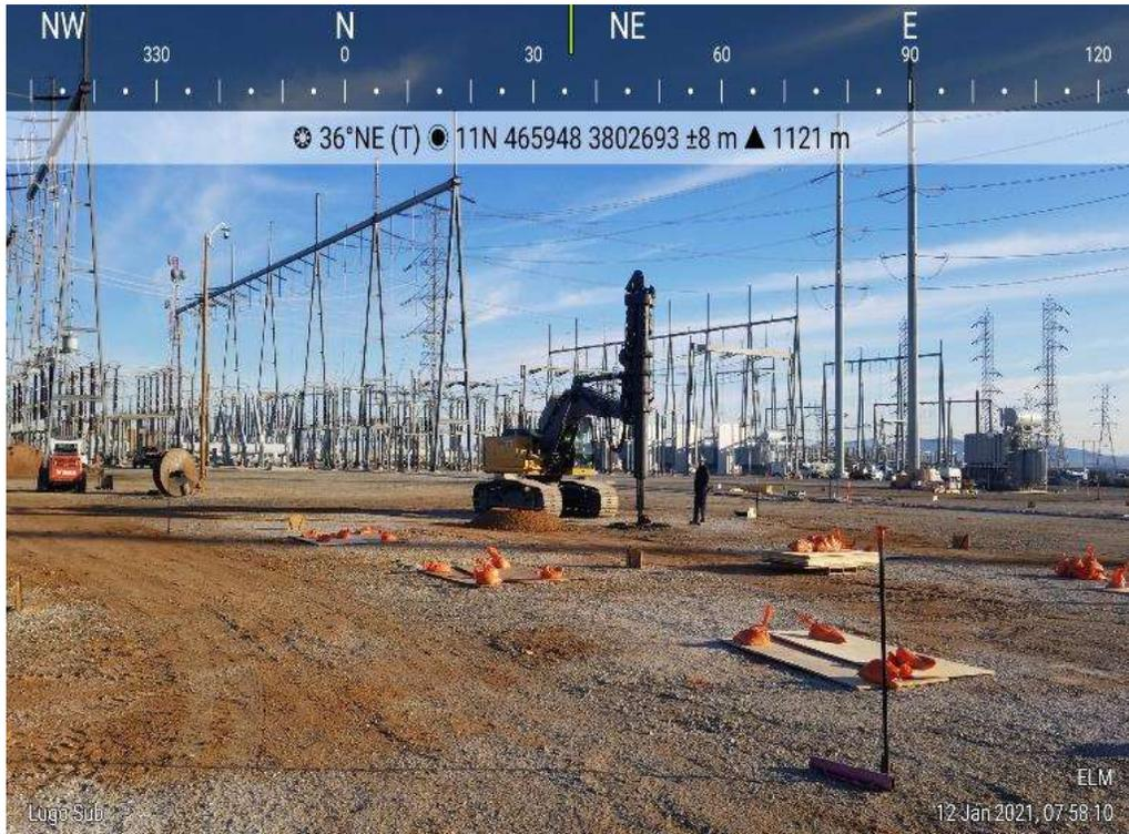
**Photo 3:** Foundation drilling occurring at the Lugo Substation (photo courtesy of SCE; January 12, 2021).
