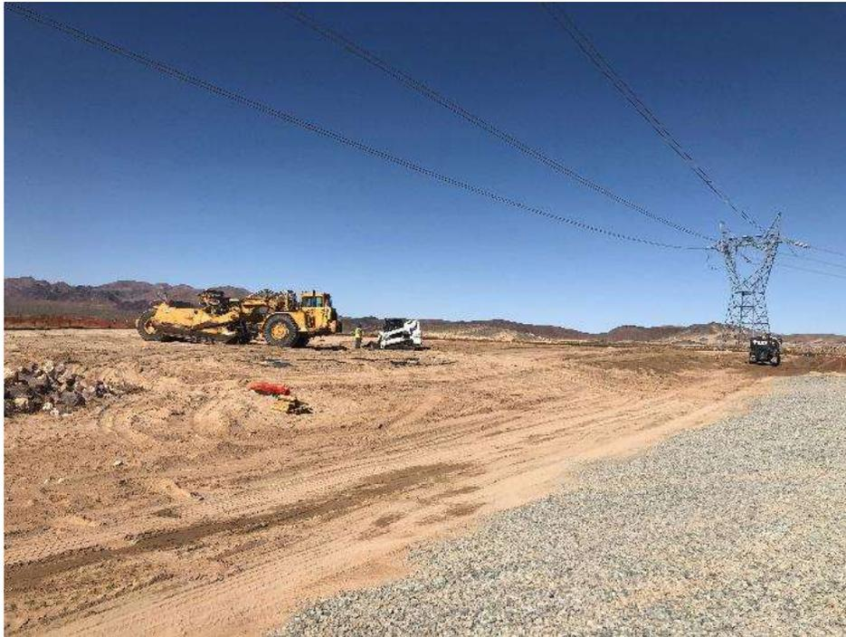
**Photo 3:** Grading at Ludlow Series Capacitor. March 30, 2021.
