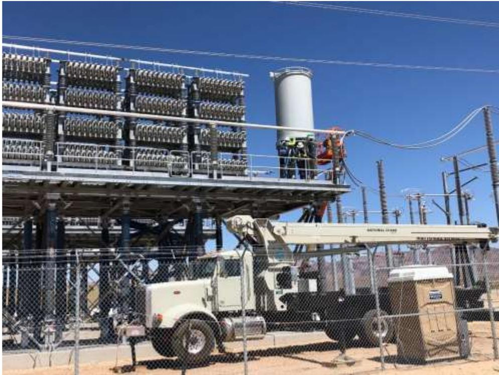
**Photo 5:** Capacitor installation at Ludlow Midline (April 13, 2022).
