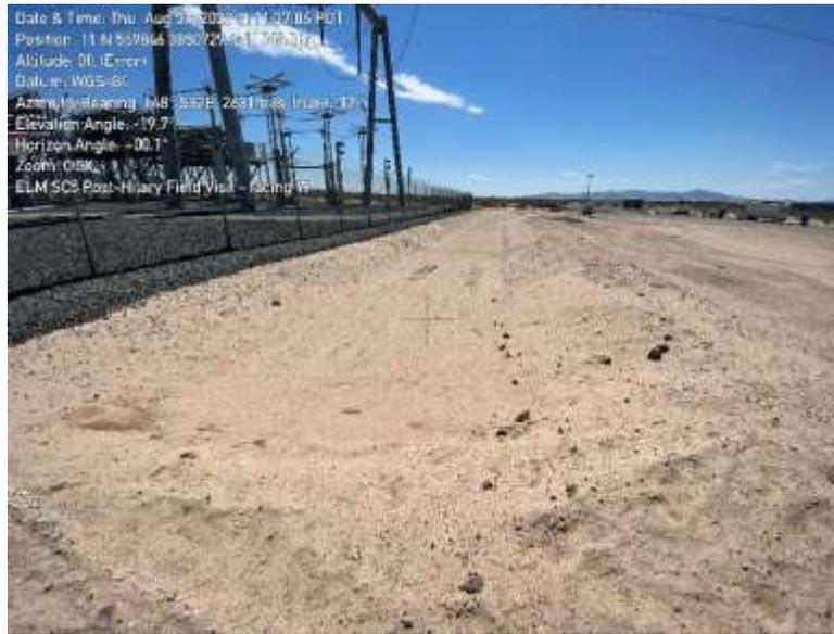
**Photo 3:** Post-Hurricane Hilary conditions at SC5. No erosion or storm damage observed along the capacitor's southern-border drainage/V-ditch (pictured, facing SW).
