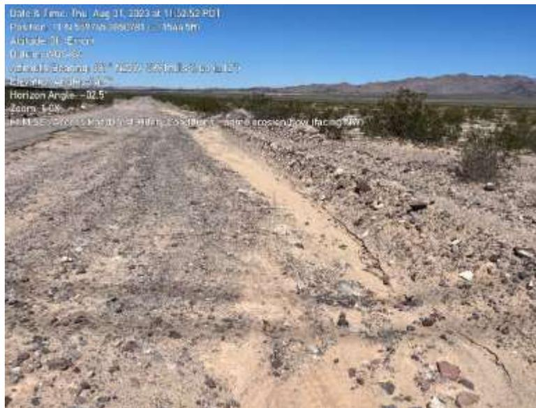
**Photo 4:** Post-Hurricane Hilary access road conditions, directly south of SC5 (facing NW). Some mild erosion observed, but erosion was not a significant-enough level to negatively affect driving conditions or pose safety risks to site personnel.
