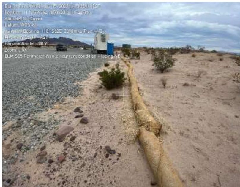
**Photo 2:** Perimeter wattle along southeastern border of SC5 deteriorating and remains in need of maintenance/repair, as noted in the weekly environmental compliance reports (SWPPP section).
