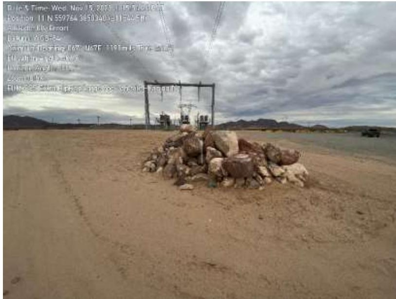
**Photo 3:** Excess large rock/riprap present on site at SC5. The intended use/purpose of this material is unknown at this time but may be leftover from SWPPP BMP-related install (berms surrounding SC5 switching station).
