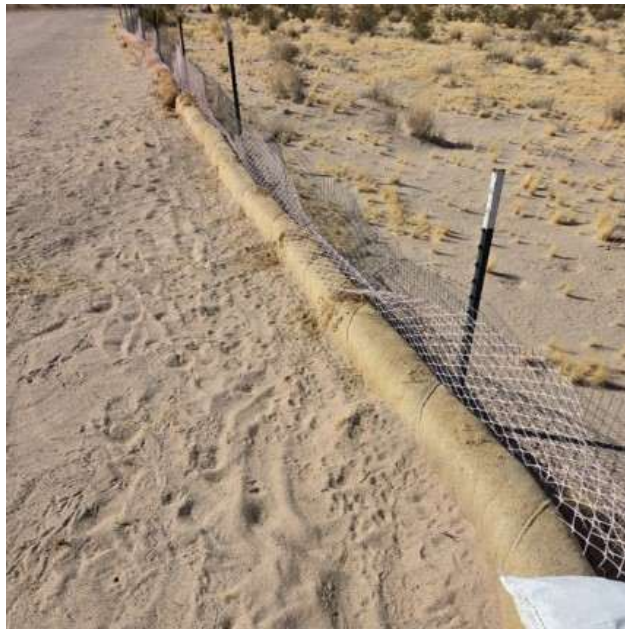
Photo 6: Replacement of deficient/damaged perimeter wattles with new/refurbished, temporary wattles at SC5 during reclamation. Photo curtesy of the October 22, 2024 QSP SWPPP inspection.
