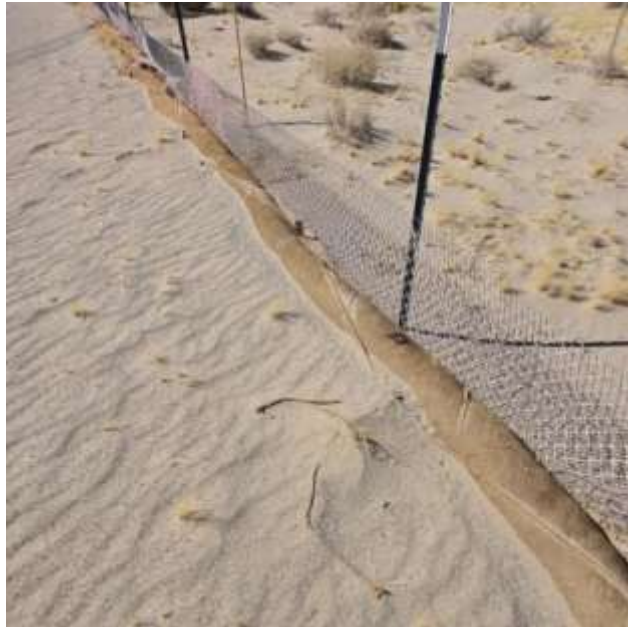
Photo 5: Significant sand accumulation/build-up, exceeding the 50% burial limit at perimeter wattles at SC5. Photo curtesy of the October 1, 2024 QSP SWPPP inspection.
