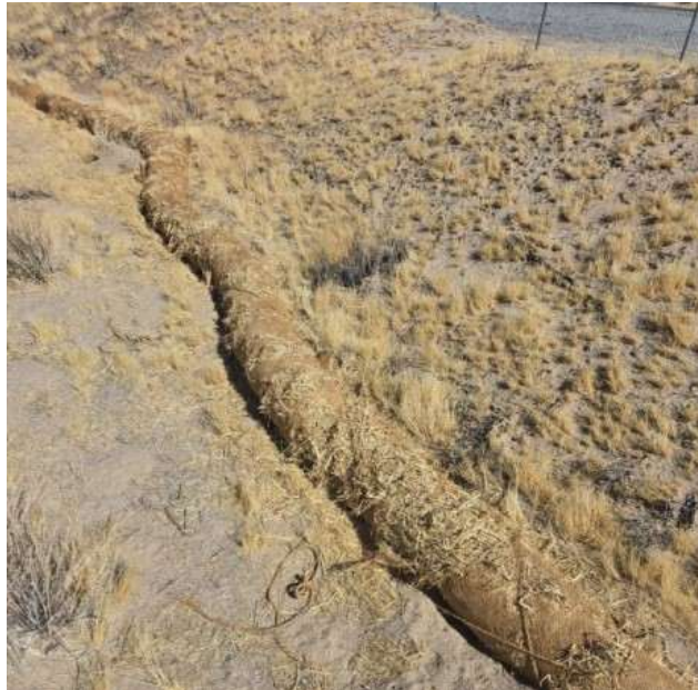
Photo 4: Damage to perimeter wattles at SC5, with a splits in the burlap covering, spill out of straw material, and loss of functionality as a BMP. Photo curtesy of the October 1, 2024 QSP SWPPP inspection.
