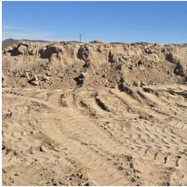
Photo 7: Removal of damaged stockpile coverings and spreading of stockpiled material during reclamation work at SC2. Photo courtesy of the October 31, 2024 QSP SWPPP inspection.
