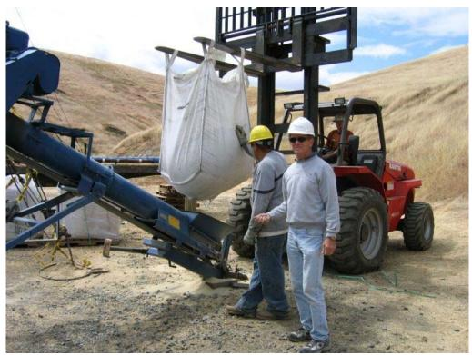
Figure 3 – System to shoot engineered sand down well, June 13, 2006
