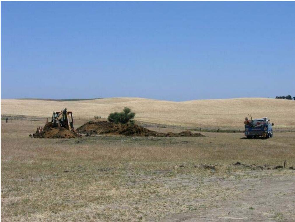
**Figure 7** – PG&E working adjacent to metering station and tapping into 32-inch existing natural gas line to supply LGS with natural gas for storage, June 19, 2006.
