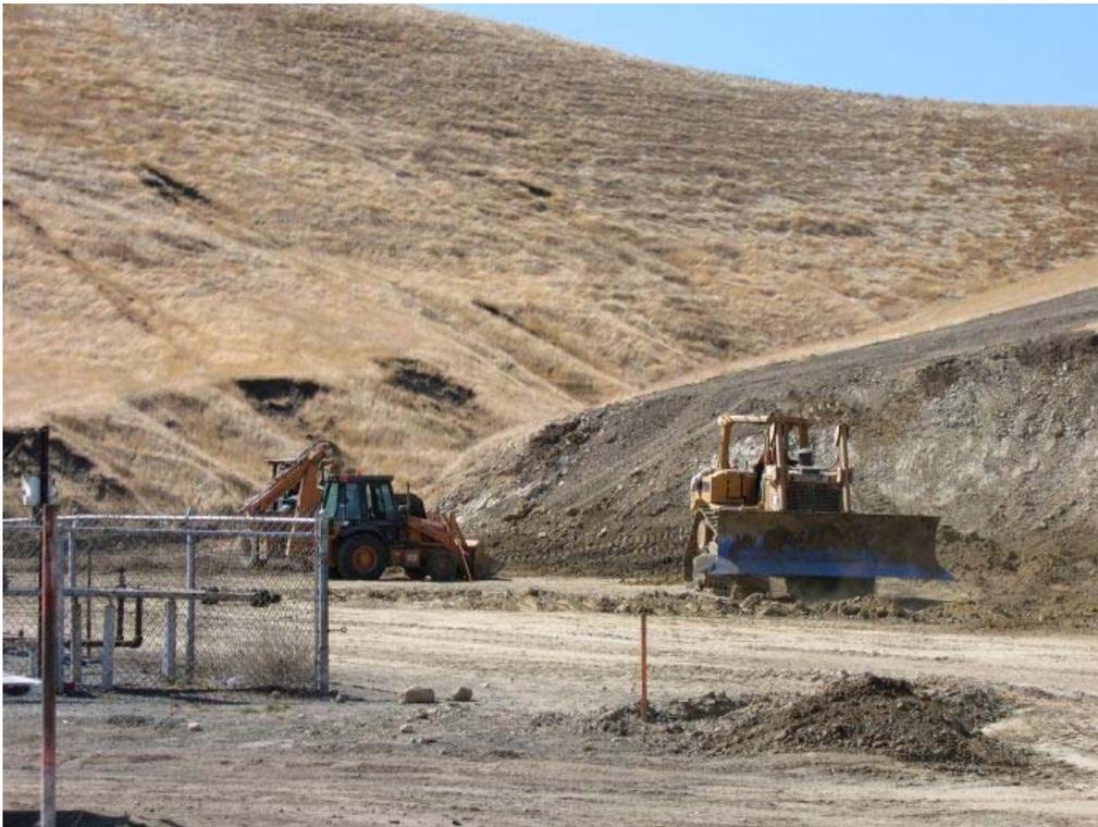
**Figure 2** – Crews backfilling pipe trench at well site S-2, September 7, 2006
