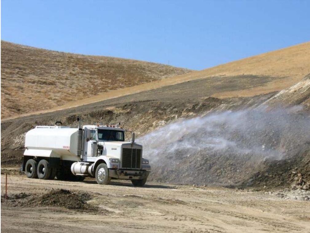
**Figure 1** – Watering work area at S-2 well site, September 7, 2006
