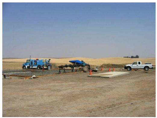
**Figure 3** – PG&E crews at the Metering Station hydrotesting the pipeline, September 12, 2006.
