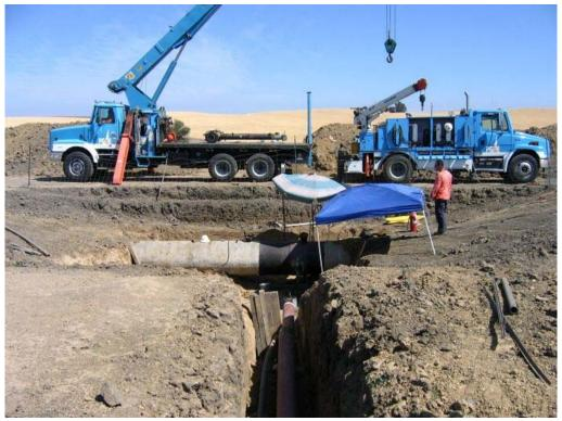
**Figure 5** – PG&E working at Metering Station conducting preparation work to tap into their 32-inch gas line, September 19, 2006.
