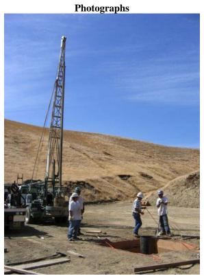
**Figure 1** – S-2 Well Site - Crews drilling pilot hole for new well, September 19, 2006
