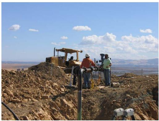
**Figure 2** – Crews conducting hydrostatic testing of pipe at Well Site S-5. October 4, 2007.
