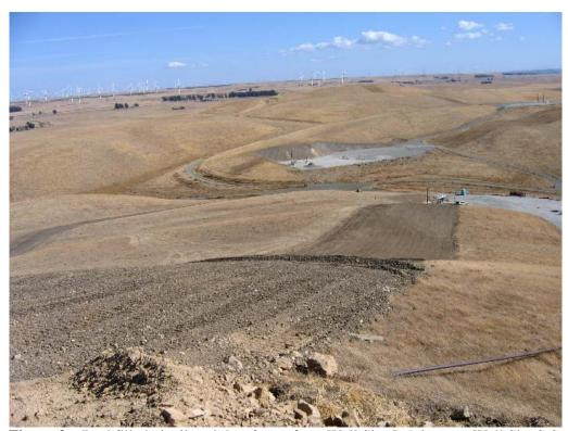
**Figure 3** – Backfilled pipeline right-of-way from Well Site S-5 down to Well Site S-2. October 4, 2007.
