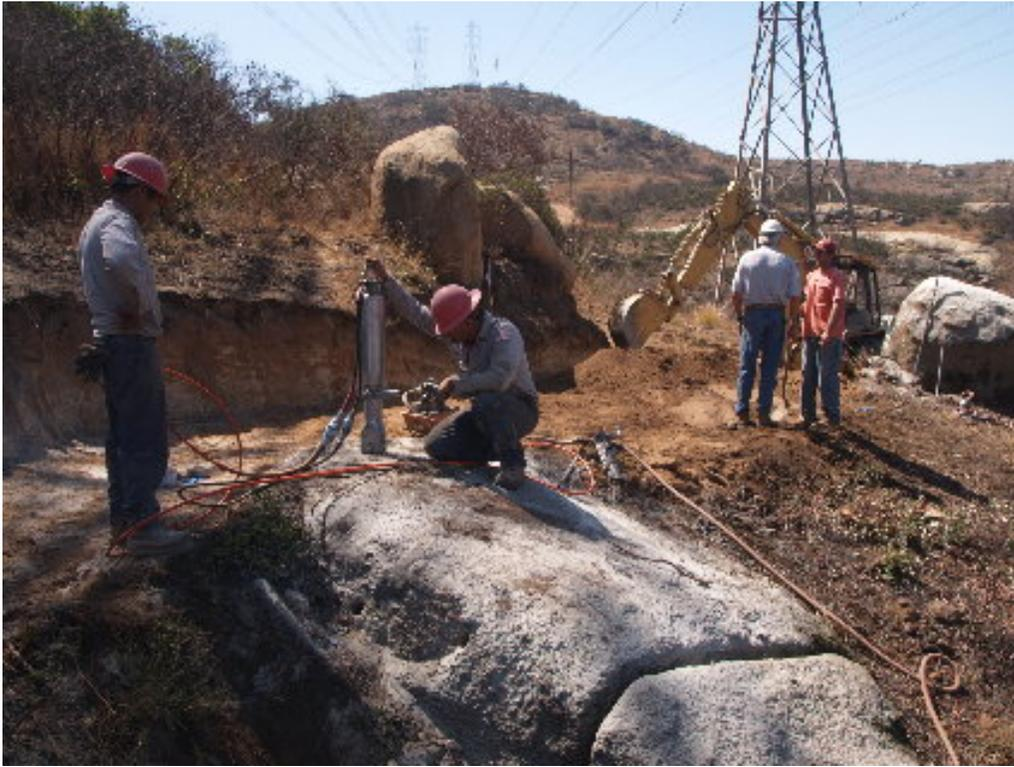
**Figure 3** – A special crew worked at hydraulically splitting the boulders at Site 912.
