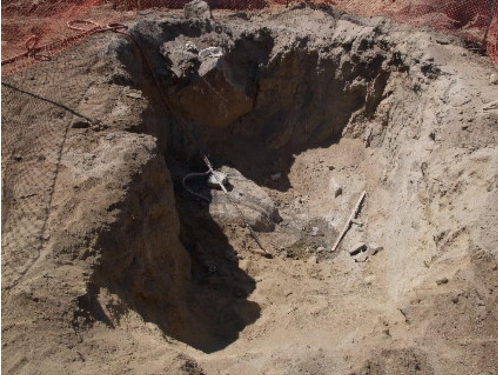
**Figure 1** – The PAR crew at Tower Site 1300 used a chemically expansive material to fracture the bedrock in the foundation hole.
