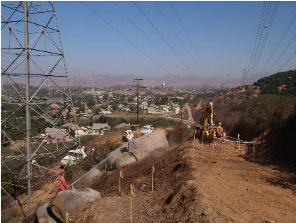
**Figure 4** – The Union crew at Site 932 worked on removing loose boulders and soil from the side slope.
