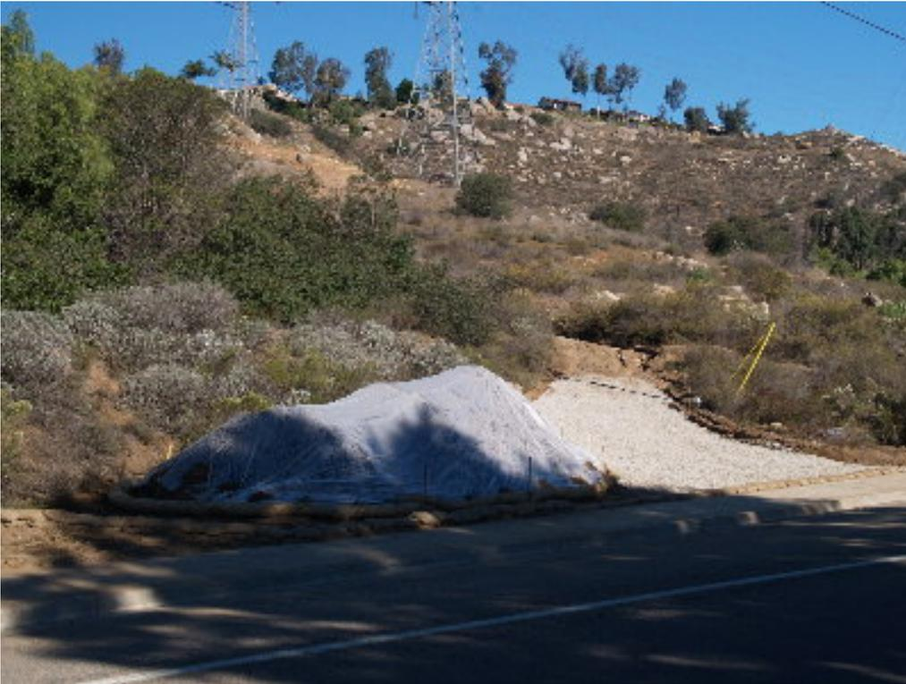
**Figure 7** – The sediment at Tower Site 440 has been cleaned from the public right-of-way and the spoil pile stabilized.
