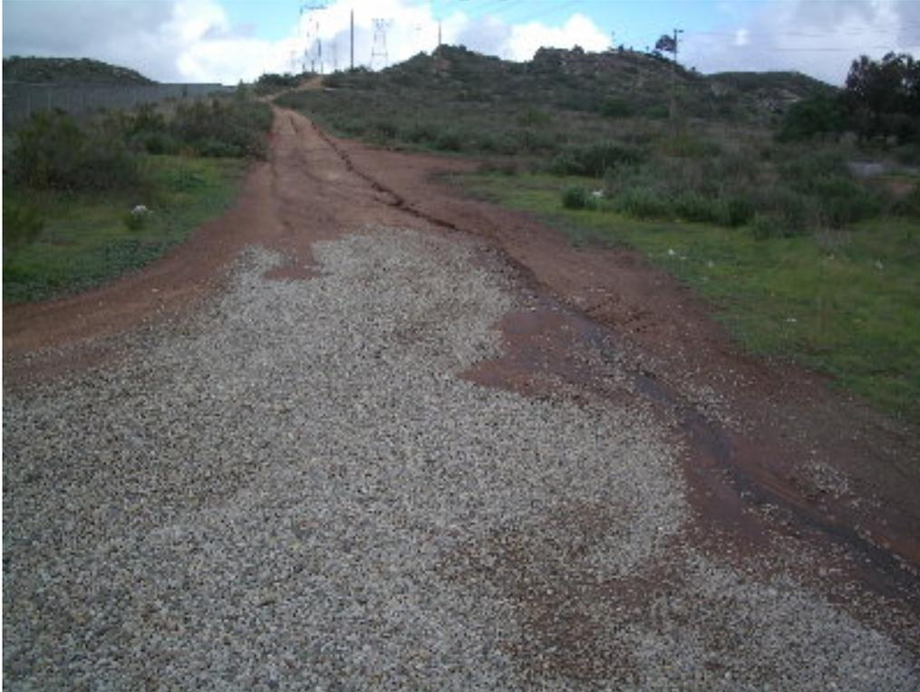
**Figure 1** – Minor erosion occurred at several access roads after recent rains. No environmental impacts were noted.
