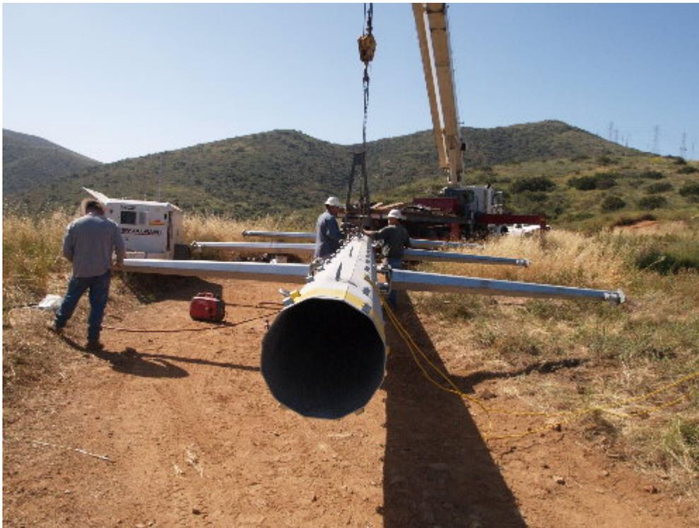
**Figure 2** – The PAR crew worked on the access road to attach the arms to the upper section of a steel pole.
