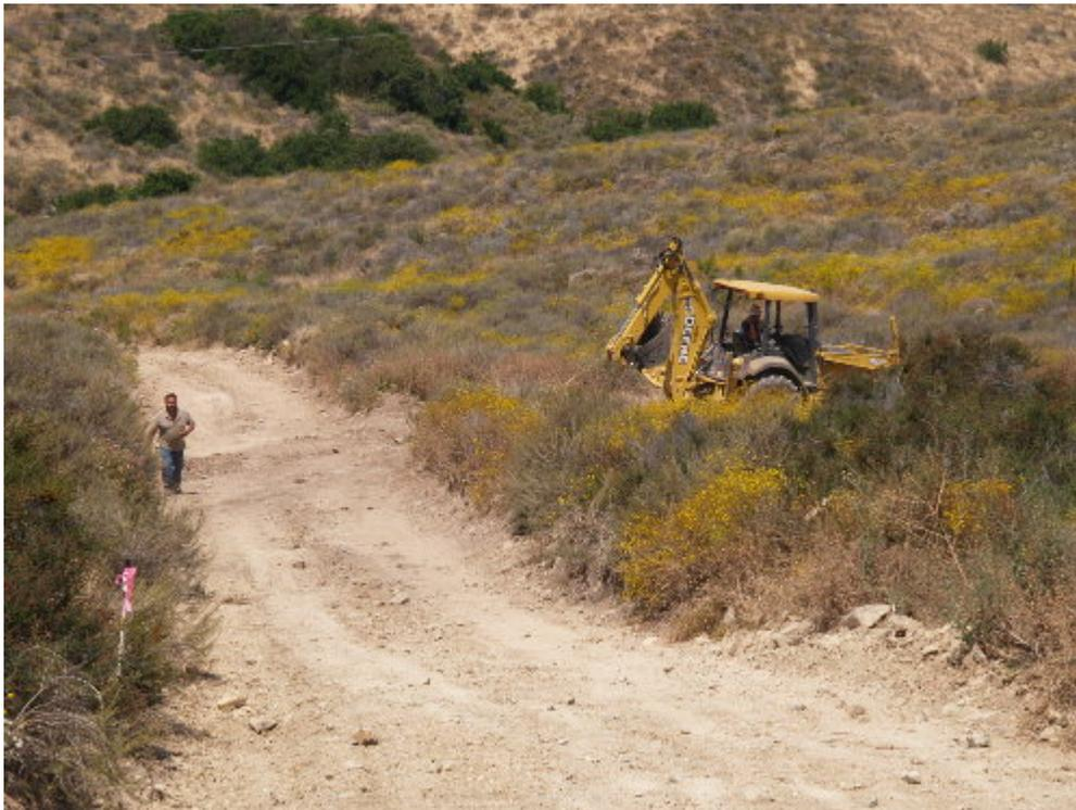
**Figure 2** – The PAR crew worked with the Essex EI to place water bars on the access road down from Pole Site 10. The backhoe is operating on an access road, not in native vegetation.
