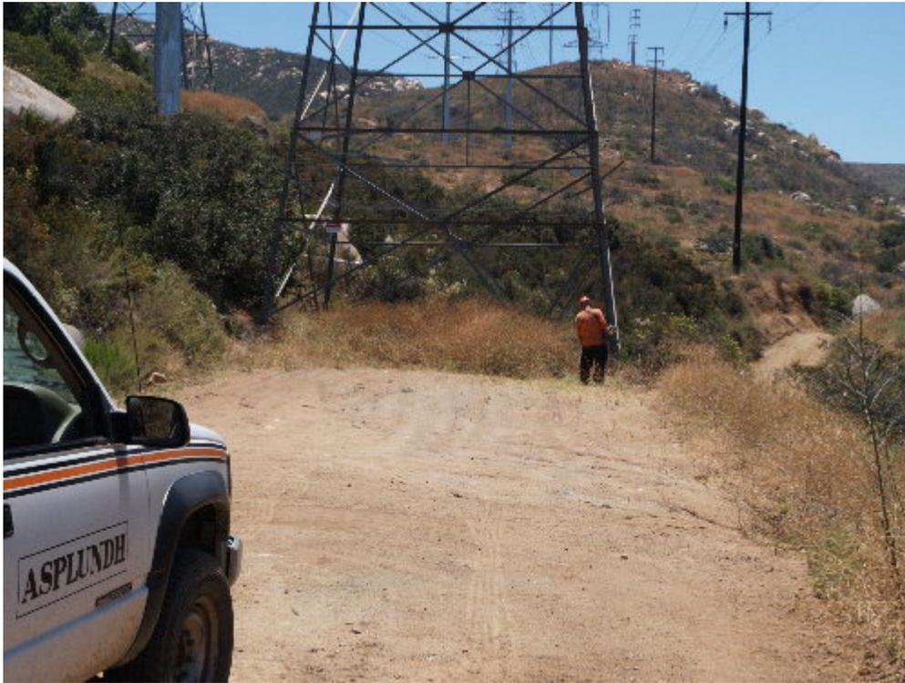
**Figure 5** – The Asplundh crew, subcontracted to Wilson, cleared ruderal vegetation from under towers in preparation for the permanent 230 kV work.
