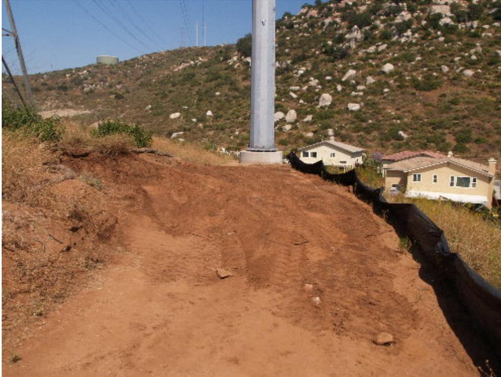
**Figure 1** – The PAR crew regraded the pad at Pole Site 1310 and placed BMPs.
