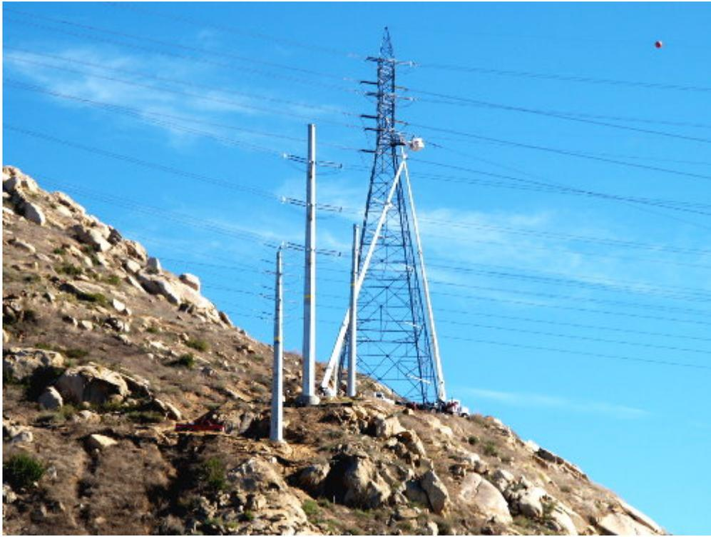
**Figure 3** – PAR crews working to replace conductor over the San Diego River span.
