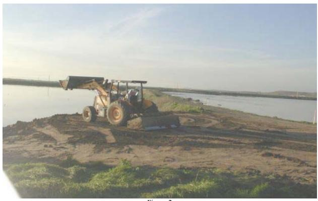
Figure 2 Creating Pole Foundation Pad #23 at the San Jose/Santa Clara Water Pollution Control Plant January 28, 2003
