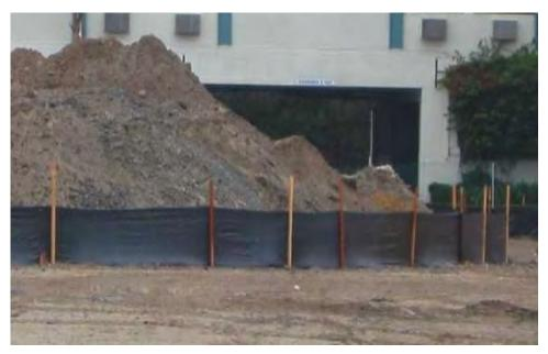
Silt fence used for stockpile perimeter control.
