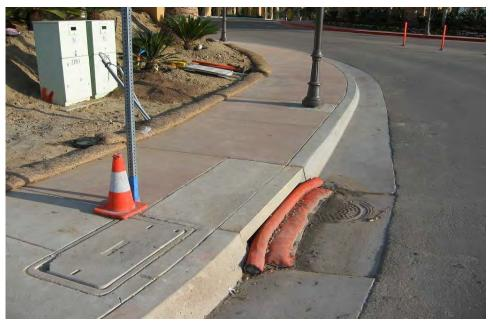
Inlet protection that blocks flow is good for preventing non-storm water discharges from entering the drain.
