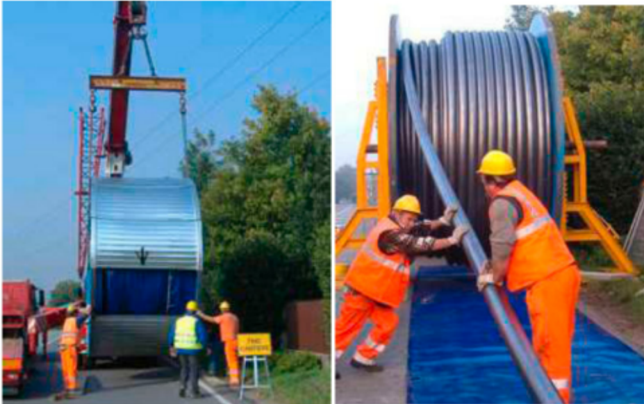
Laying operation, Tubigo near Milan 2005, Prysmian extruded cross-linked polyethylene XLPE cable
