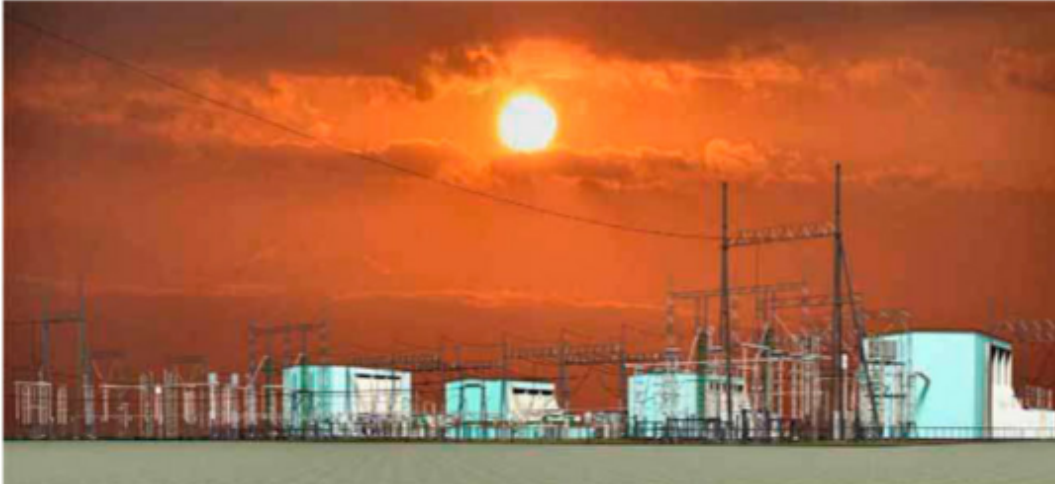
+/- 800 kV 6400 MW DC converter station
