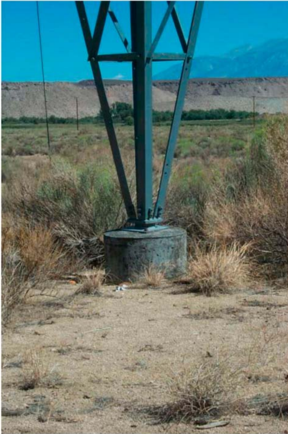
Pylon foundation, Pacific Intertie 3,100 megawatts, 1965 LADWP
