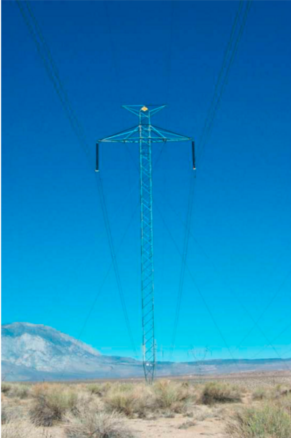
Pacific Intertie 3,100 megawatts, +/-500 kV DC, 1965 LADWP
