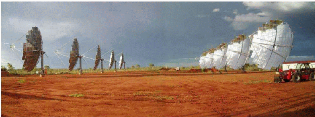
154 megawatt solar concentrator power station in Victoria Australia, at the higher cost of $2.70 per watt, potentially located on a farm, (solarsystems.com).
