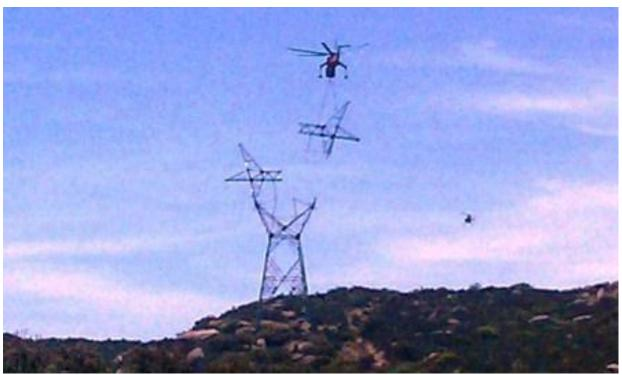
Aircrane delivering pre-assembled tower piece at Tower EP83, Link 2.
