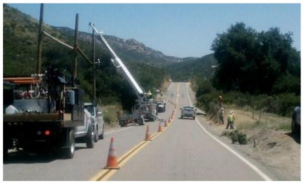
Guard structure installation on Lyons Valley Road near Tower EP24. (Link 2)
