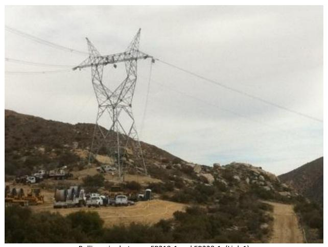
Pulling wire between EP219-1 and EP220-1. (Link 1)
