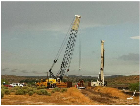
Drilling and caisson hammering at EP240, Link 1.
