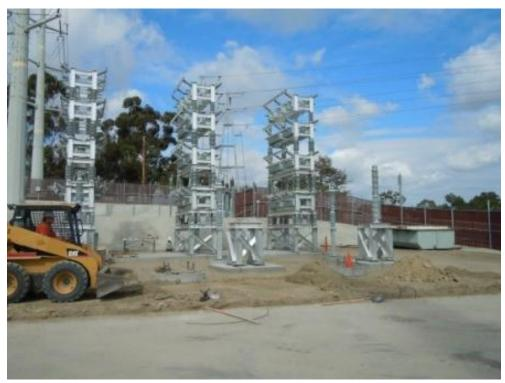
Installation of capacitor bank at San Luis Rey Substation.
