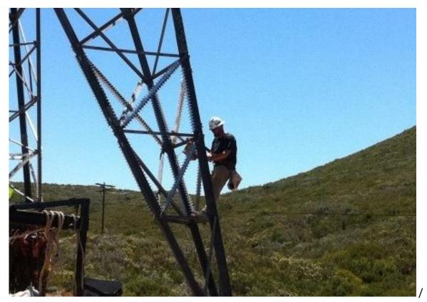
Installing anti-climbing guards at EP27-1. (Link 2)
