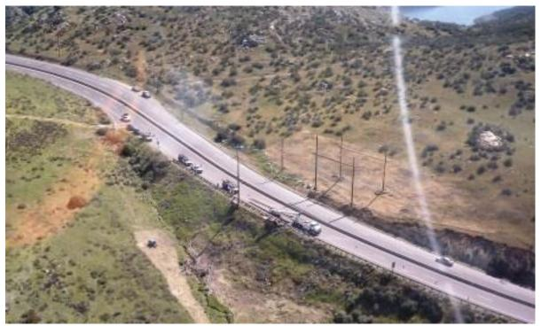
Installation of guard structures across Highway 67 near EP36. (Link 5)
