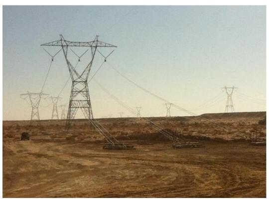
Wire and snubs at EP322 EP323 pull site. Temporary mats have been removed. (Link 1)
