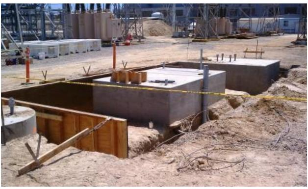
Wood work for pouring concrete foundation at Encina Substation.
