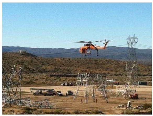
Aircrane "picking" a pre-assembled tower piece for Tower EP228.
