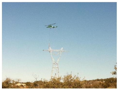
Insulator installation at EP217, Link 1.
