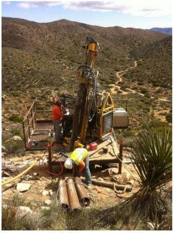
Micropile drilling at EP 225-1, Link 1.
