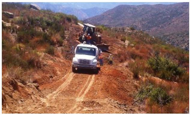
Grading operations on access road to EP40-1. (Link 2)
