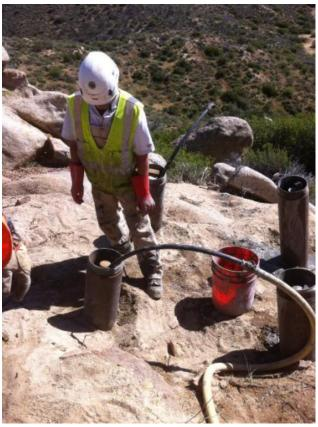
Micropile grouting at EP 225 1, Link 1.
