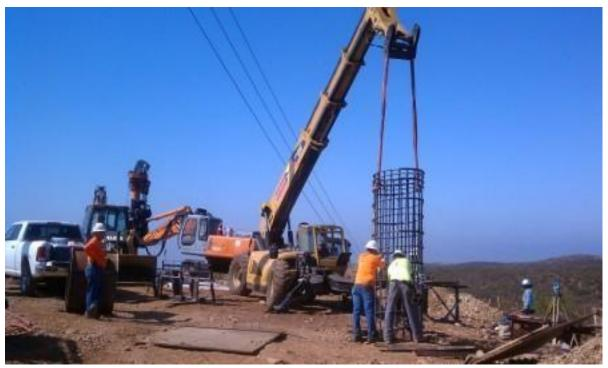
Installation of rebar at CP19-1, Link 5.
