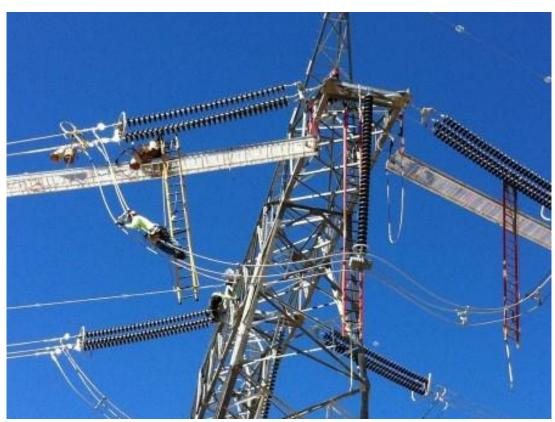
Installing jumpers at Tower EP200-3. (Link 1)
