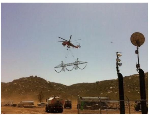
Aircrane flying tower bridge to Tower EP54. (Link 2)
