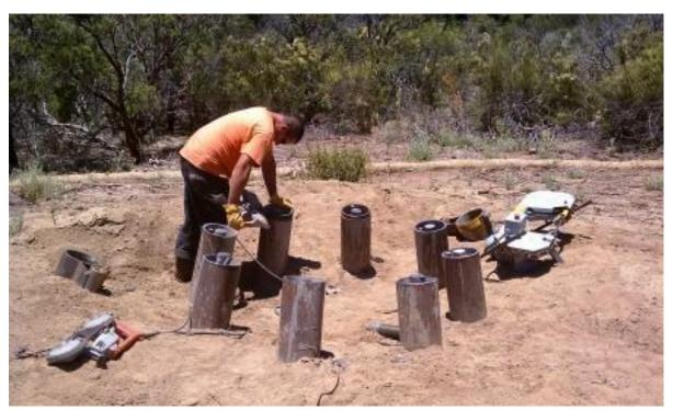
Trimming micropiles at EP 85-2, Link 2.
