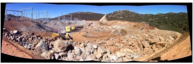
Rock being crushed for Class 2 base and select fill. (Link 3)
