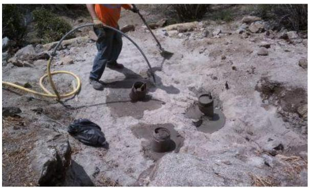
Micropile grouting at Tower EP 81, Link 2.
