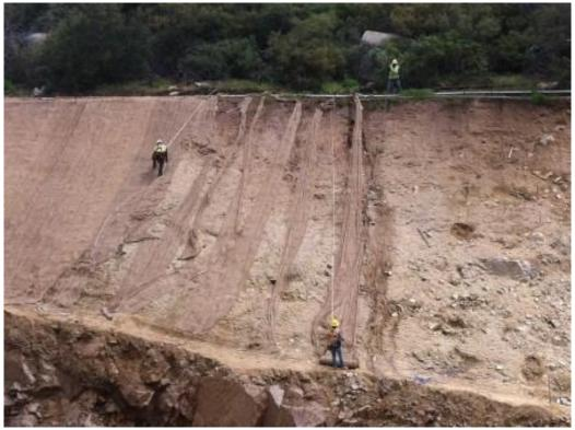
Jute installation along cut slopes at Suncrest Substation. (Link 3)
