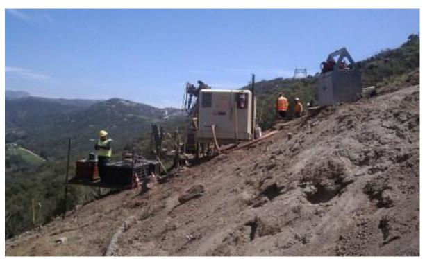
Micropile drilling at EP10-2, Link 2.
