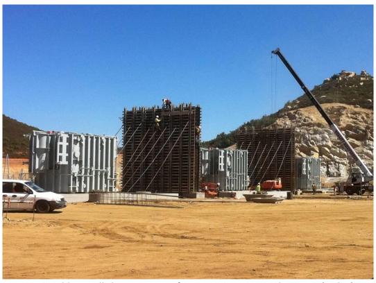
Forming blast walls between transformers at Suncrest Substation. (Link 3)
