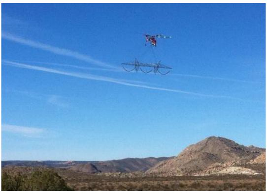
Aircrane flying bridge to EP253-3. (Link 1)
