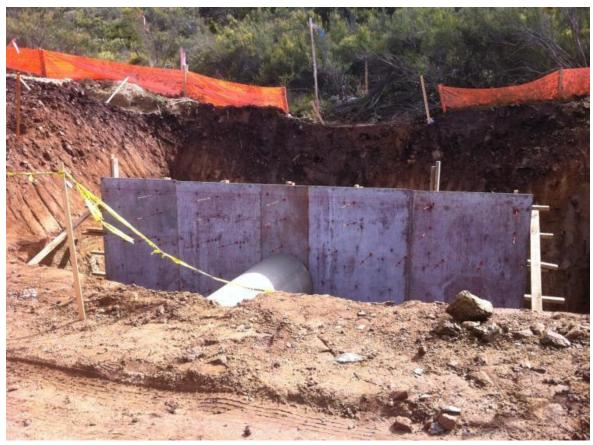
Culvert installation along BBTT, Suncrest Substation, Link 3.
