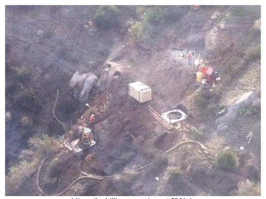
Micropile drilling operations at CP61-1.
