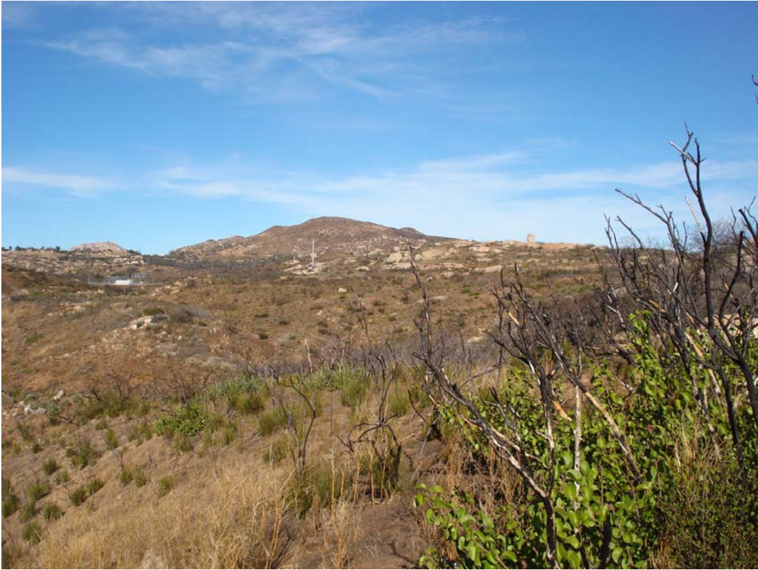
Looking at Barrett Substation
