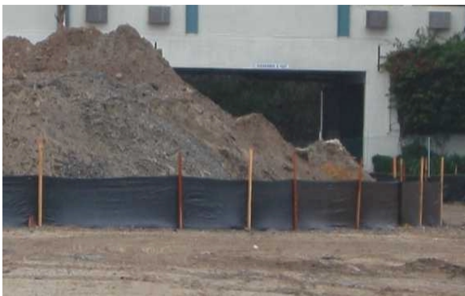
Silt fence used for stockpile perimeter control.
