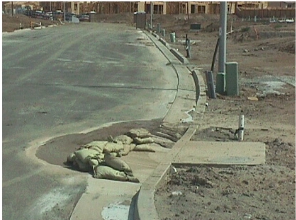
Gravel bag inlet protection.
