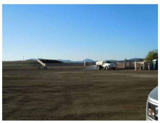
Figure 5: Water truck performing dust control activities at the Alpine Laydown Yard.
