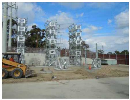
Figure 1: Installation of capacitor bank at San Luis Rey Substation.
