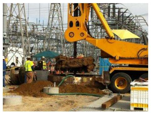
Figure 3: Foundation drilling for 230 kV termination pier at Encina Substation.
