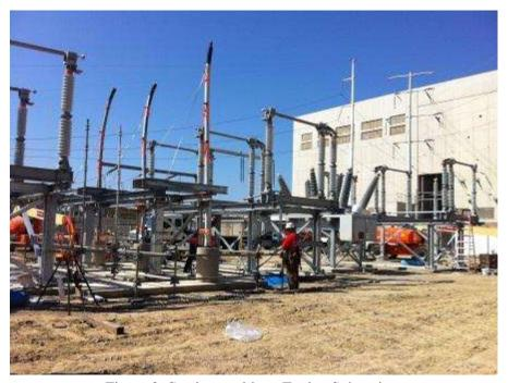
Figure 2: Steel assembly at Encina Substation.
