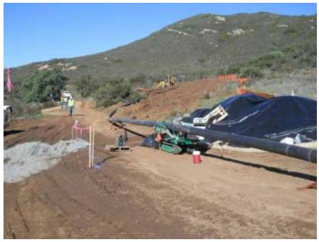
Figure 3: Above ground water line assembly at Suncrest Substation.
