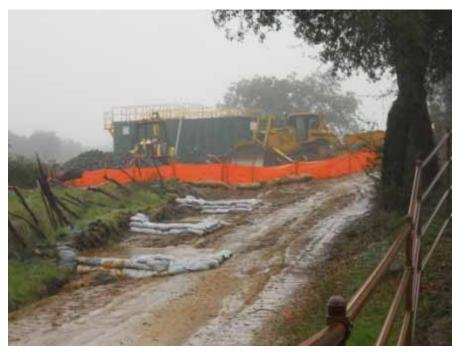
Figure 4: BMPs at Suncrest Substation during rain event.
