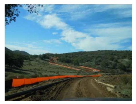
**Figure 3**: Vegetation clearing, rough grading and waterline installation at the Suncrest Substation.
