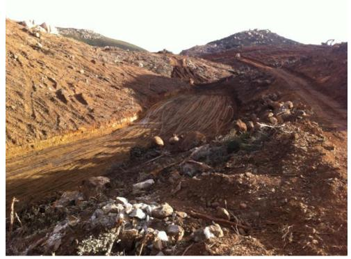
**Figure 5:** Sediment basin construction, Link 3.
