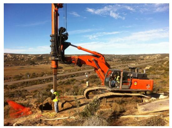
**Figure 1:** Foundation drilling at EP 219, Link 1.
