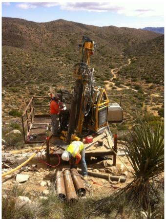
**Figure 3:** Micropile drilling at EP 225-1, Link 1.
