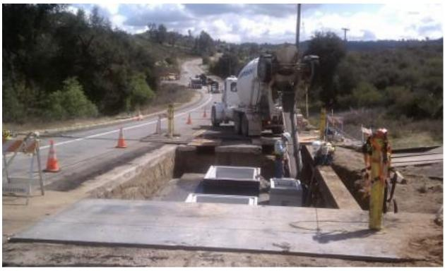
Figure 5: Concrete being poured at Vault 2L, Link 4.
