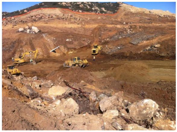
**Figure 5:** Grading and drain installation in southern portion of the Suncrest Substation pad site, Link 3.
