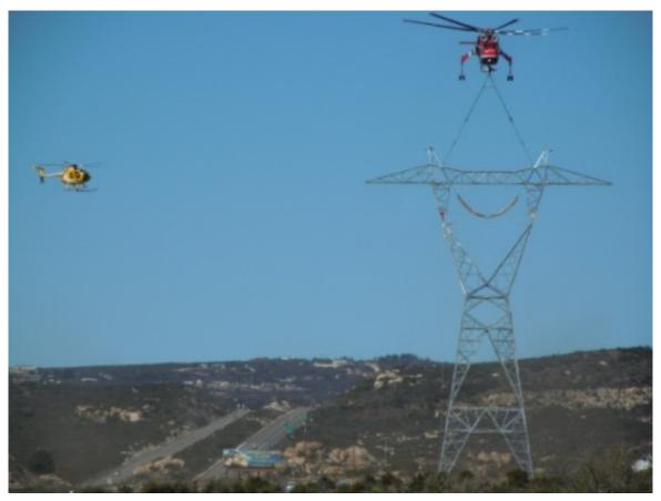
**Figure 1:** Air crane is placing the bridge on EP 217, Link 1.
