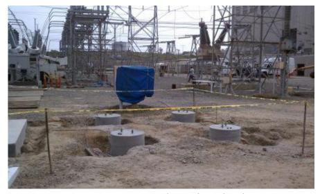
**Figure 7:** Footers poured at Encina Substation.
