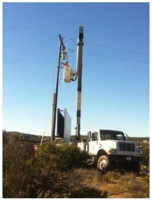
**Figure 2:** 12 kV relocation along McCain Valley Road, Link 1.
